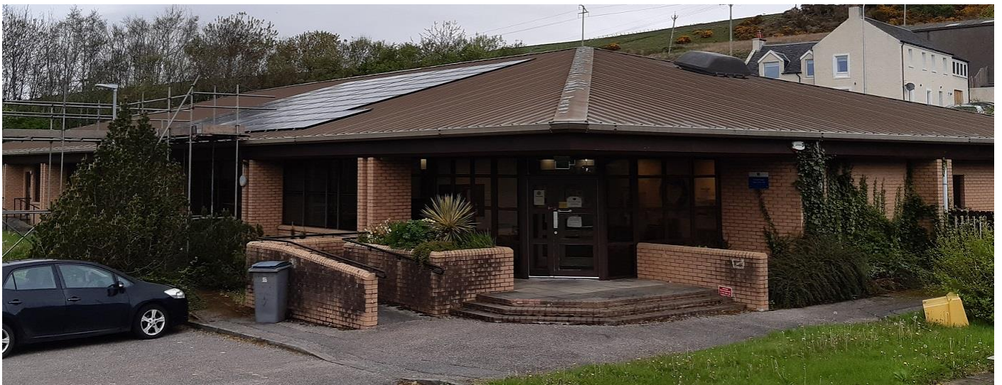
Image of Solar PV at Kintyre House, Campbeltown.
