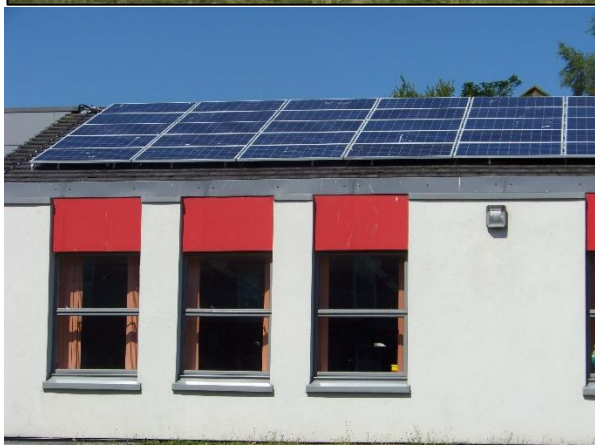
Image of off-site manufactured biomass boiler-house installed at Ardrishaig Primary School and some of the roof mounted solar pv panels installed at Hermitage Primary School in Helensburgh.
